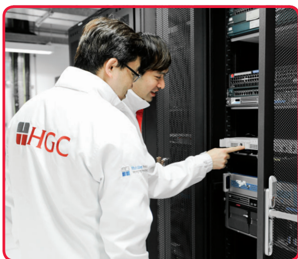
HGCGC provides world-class data centre facilities for customer organisations throughout a variety of industries.
