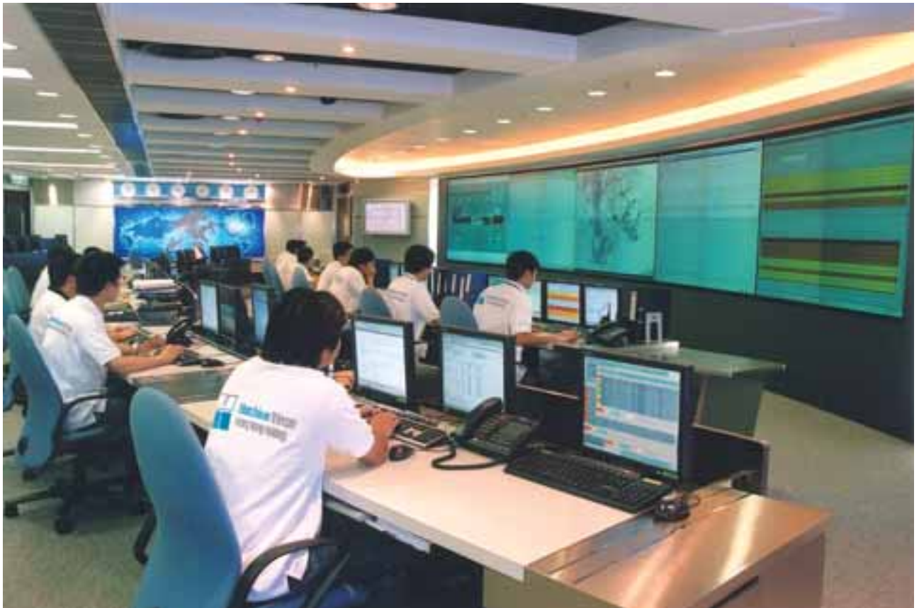
• 3 Hong Kong's Central Network Control Centre ensures the highest level of mobile network performance
